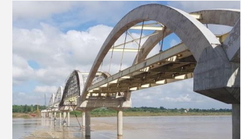
179,845 kms of temporary bridge upgrades
