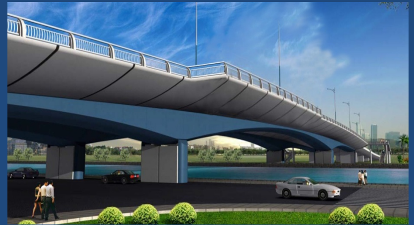
Bridges in Pasig
