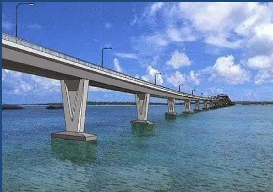
Panguil Bay Bridge
